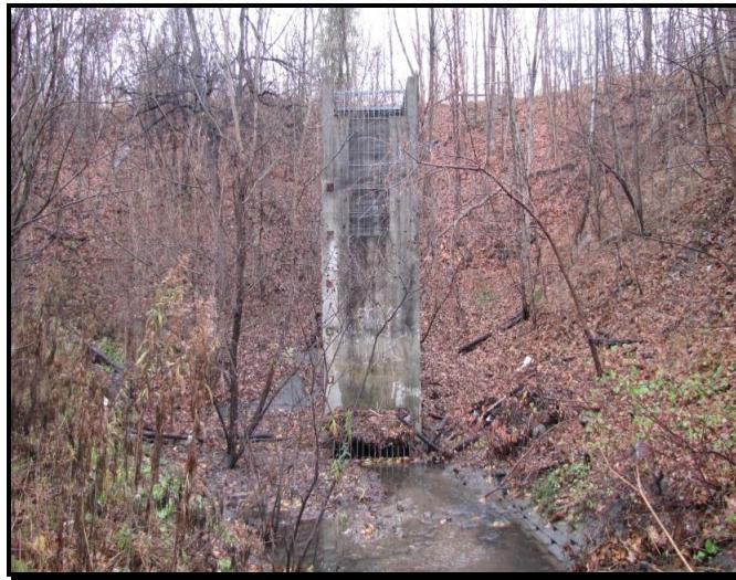
**Figure 2-18: Water level markings on outlet structure – Conlins pond**
