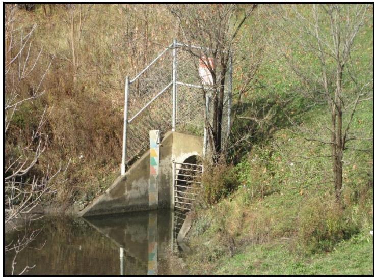
**Figure 2-19: Water level markings on inlet structure – Malvern 10A pond**
