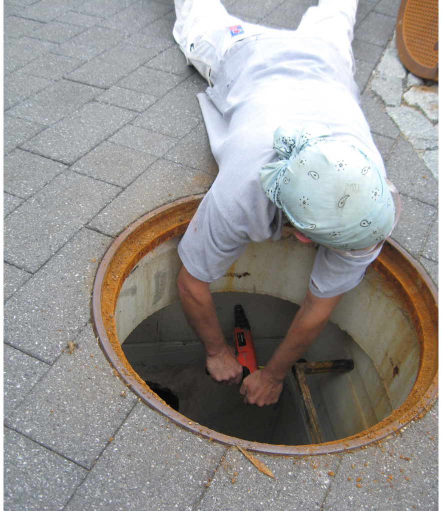
Figure 25. Installation of the Pressure Transducers at the Overflow of the Cistern (Credit: Emily McCoy)
