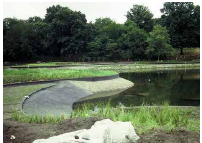
Figure 50. Planting the marsh soils around Belvedere Lake in Central Park, NY, NY
