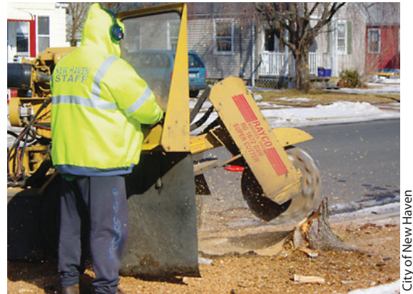
Figure 8: Tree-Stump Removal
