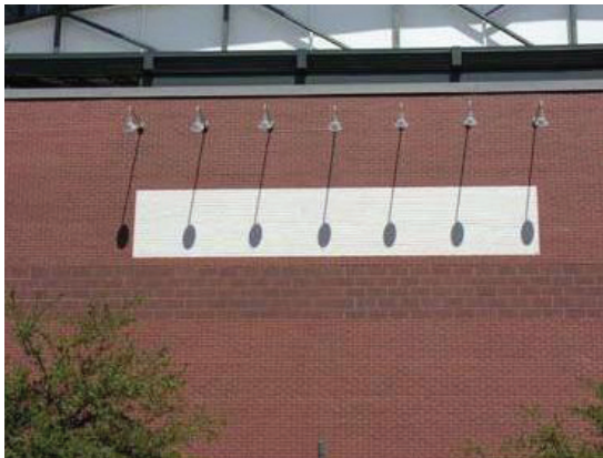
Albedo alone can significantly influence surface temperature, with the white stripe on the brick wall about 5–10°F (3–5°C) cooler than the surrounding, darker areas.
