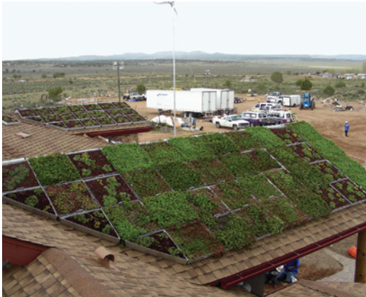
This home in Arizona shows a modular green roof on a steep-sloped roof.
