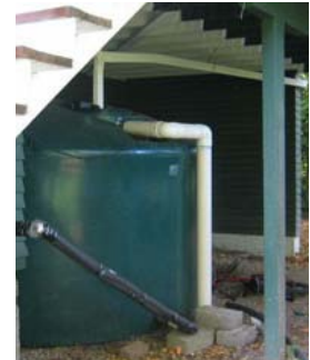
Cistern located under a porch
