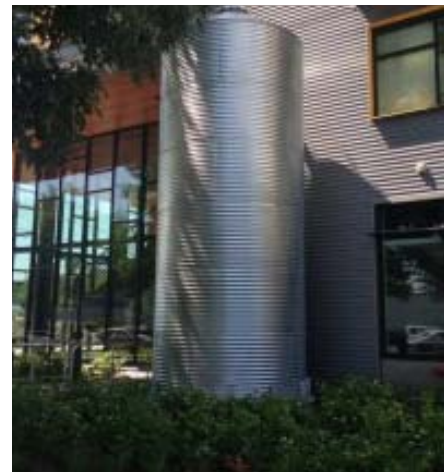
Cistern that complements the industrial character of a development
