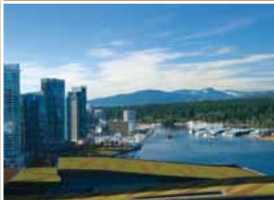
Cover Image: The Vancouver Convention Centre expansion features a 6.5 acre living roof. Photo courtesy of the Vancouver Convention Centre.
