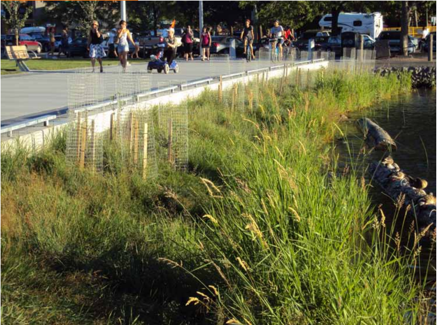
Foreshore restoration. Terry Klassen, MBCSLA.
