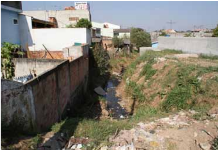
Vila Ulisses existing condition.
