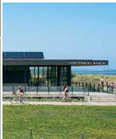
Cover Image: New facilities at Centennial Beach – Boundary Bay Regional Park. Image courtesy of eta landscape architecture inc.
