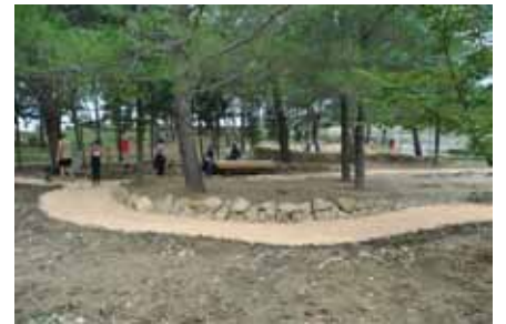
Major hardscape elements - The pier, traditional dry stone walls, and a pathway system, start to give form to the site.
