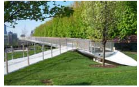
Shallow slope bridge in Millennium Park, Chicago, IL. Image courtesy of Edward K. Uhler.
