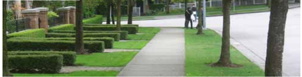
A straight, clear, path of travel with an even concrete surface. The landscaping offers wayfinding cues and acts as a buffer between pedestrians and motor vehicles. Image courtesy of Heather McCain. Please see insert for more images.
