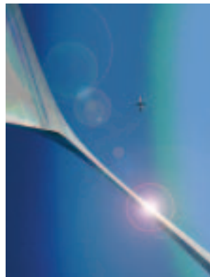
The Gateway Arch in St Louis was designed in 1947 by Eero Saarinen and built from 1961 to 1965. It still feels contemporary today. The mathematical precision of its design and construction is inspiring, given that : a) no computers were used, b) it is a catenary curve, c) it had to be built from two points and meet precisely at its apex, by old school survey, without lasers, d) it has a tapering cross section from a fifty-four foot equilateral triangle at base, rising to seventeen feet at apex and e) it was not self supporting until the two sides of the arch were connected with keystone pieces and during construction each leg had a large creeper crane, adding 100 tons to the load. Slide-rules-a-go-go.
