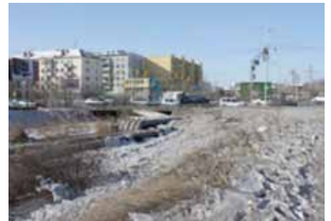
Photograph of existing condition: the channel and infrastructure. Credit: Yekaterina Yushmanova
