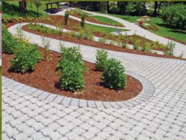
Unlike traditional asphalt or concrete, permeable pavers allow rainwater to return naturally into the ground below, reducing the concerns associated with stormwater runoff, including erosion and pollution.
