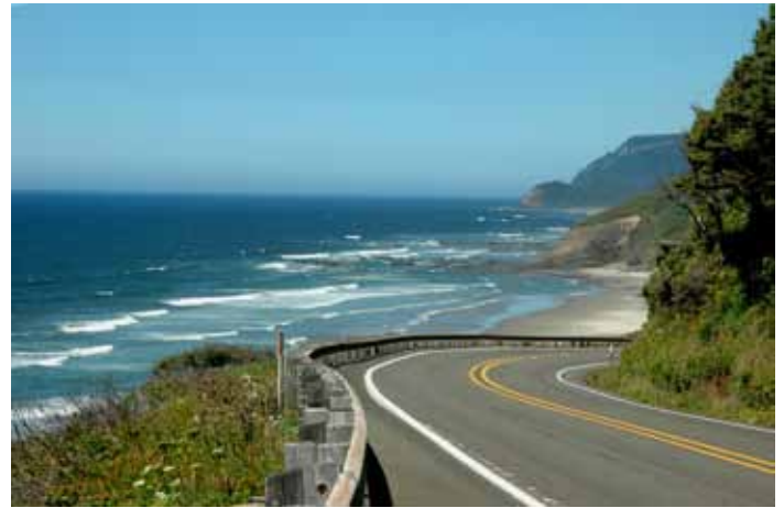
Typical Pacific coast riding conditions with shoulder improvements along the southbound lane. Image is viewing north. Image courtesy of Patrick Harrison, MBCSLA.
