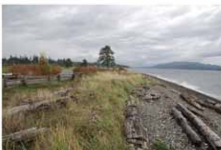
Dick Murphy Park beach restoration. Top image - as found condition, December 2004. Middle image - as constructed, March 2005. Bottom image - soft shore protection as of summer 2011. More on JPH Consultants Inc.’s softshore protection work at: http://greenshores.ca/sites/greenshores/documents/media/135.pdf . Images courtesy of Patrick Harrison, MBCSLA.
