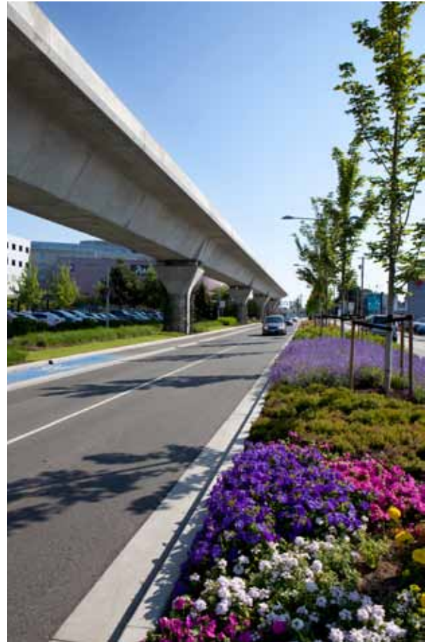
Streetscape improvements along No. 3 Road in Richmond. Credit: Canada Line
