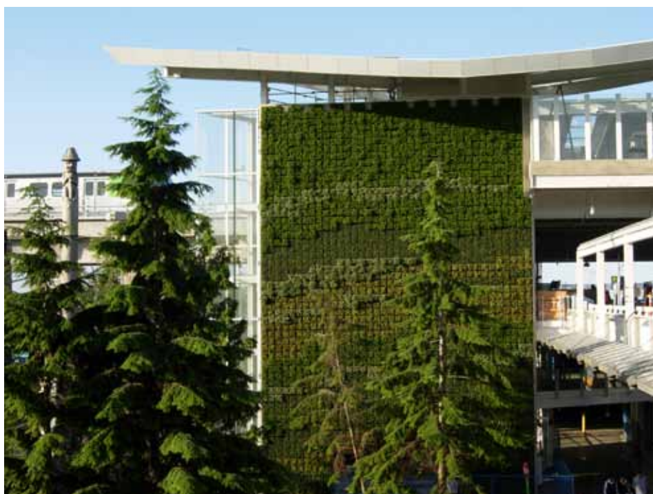
The Canada Line final stop at YVR International Airport features a 18m high green wall. Credit: Sharp & Diamond Landscape Architecture Inc.
