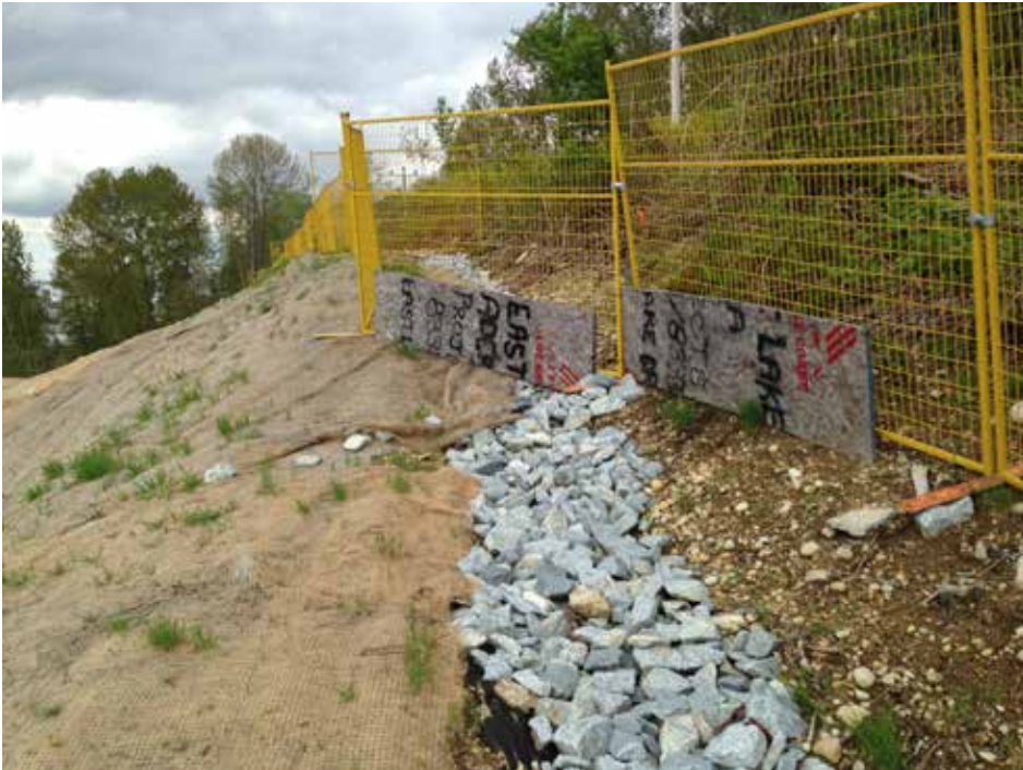
Figure 11. Swale at top of slope, waiting to be planted. Photo: Zalite
