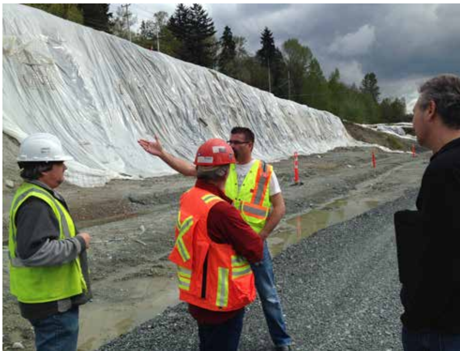
Figure 10. Consultant Team On Site – Site superintendent Dwayne Ostheidt, Landscape Architect Jonathan Losee Ltd., Blue Pine Contractor Mike Lalonde, and Geotechnical Engineer Paul Davies at the bottom of the protected slope. Photo: Zalite
