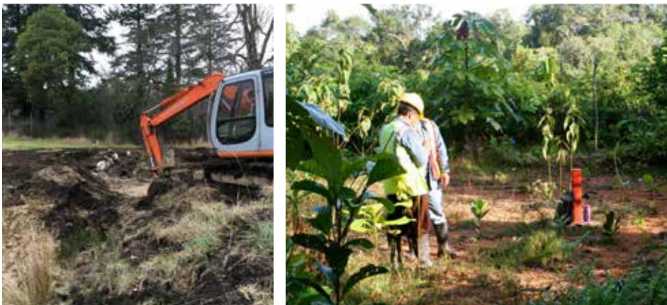
Left: Figure 2. Excavating a new stream channel for Grosbeak Creek in Saanich, BC. Photo: Strong Right: Figure 3. Re-vegetating drilling platforms in Panama. Photo: Rokosh
