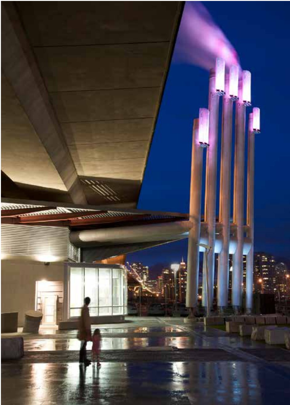
LEFT: Southeast False Creek Energy Utility Plaza PHOTO: Eckford + Associates
