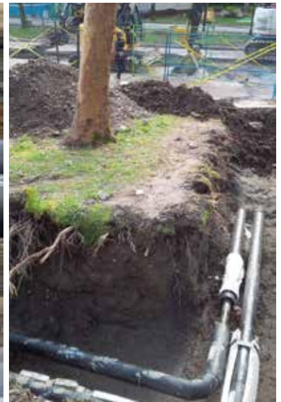
Tree roots affected by excavation for new utility infrastructure
